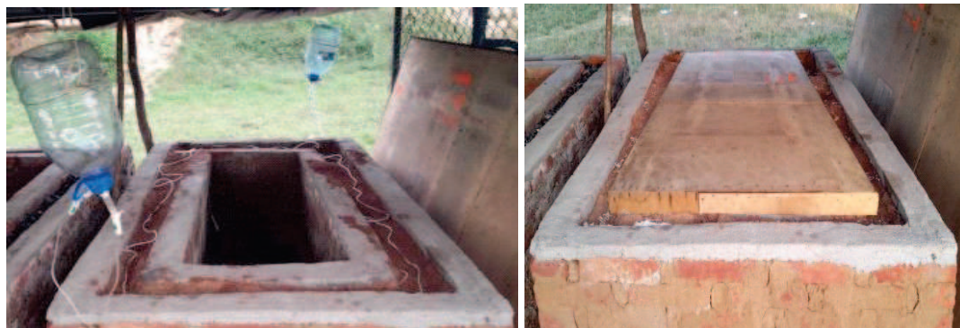
Plate 1: Fabricated double-Layer evaporative Cool-Chambers
